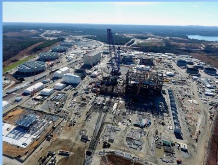
V. C. Summer 2 and 3 units under construction, South Carolina
